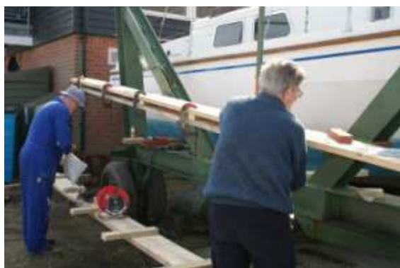
refitting the boat hoist
